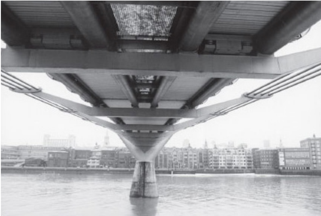
Figure 6 Close-up of the bridge's structure showing suspension cables
